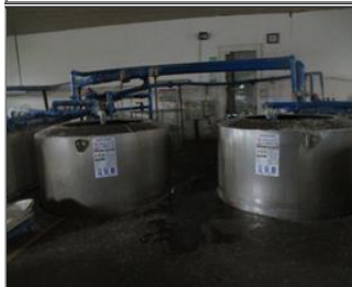
Photo of the inside of the main production hall 9. Pulping section 1.JPG
