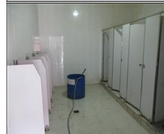
Photo of the sanitary facilities 13. Toilet.JPG
