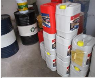
Photo of non-conformity 5. NC 7.7 No secondary container.JPG
