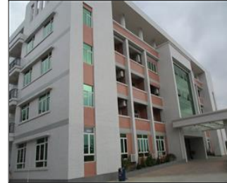
External photo(s) of the production unit(s) 1. Office building.JPG
